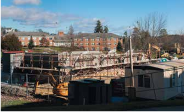
Construction scene of the Integrated Media and Studio Arts building
